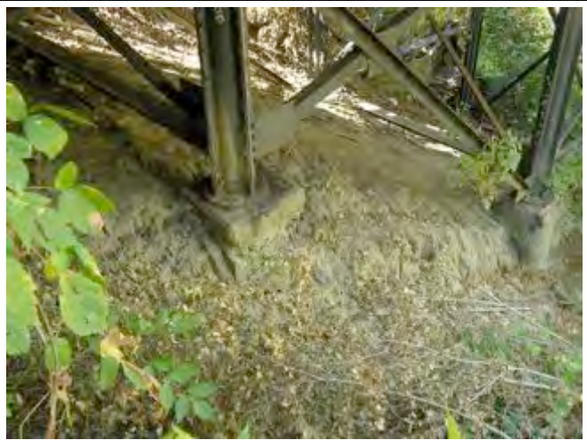
12. Erosion damage to bridge piers – Red Bank Road over Indiana and Ohio Railroad
