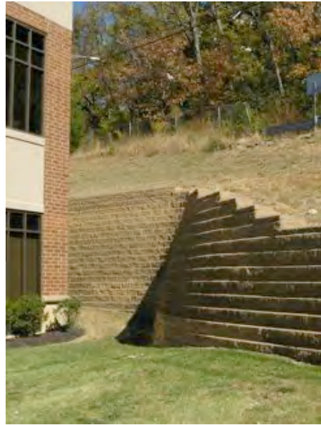
8. Existing 12 ft high retaining wall below Red Bank Road
