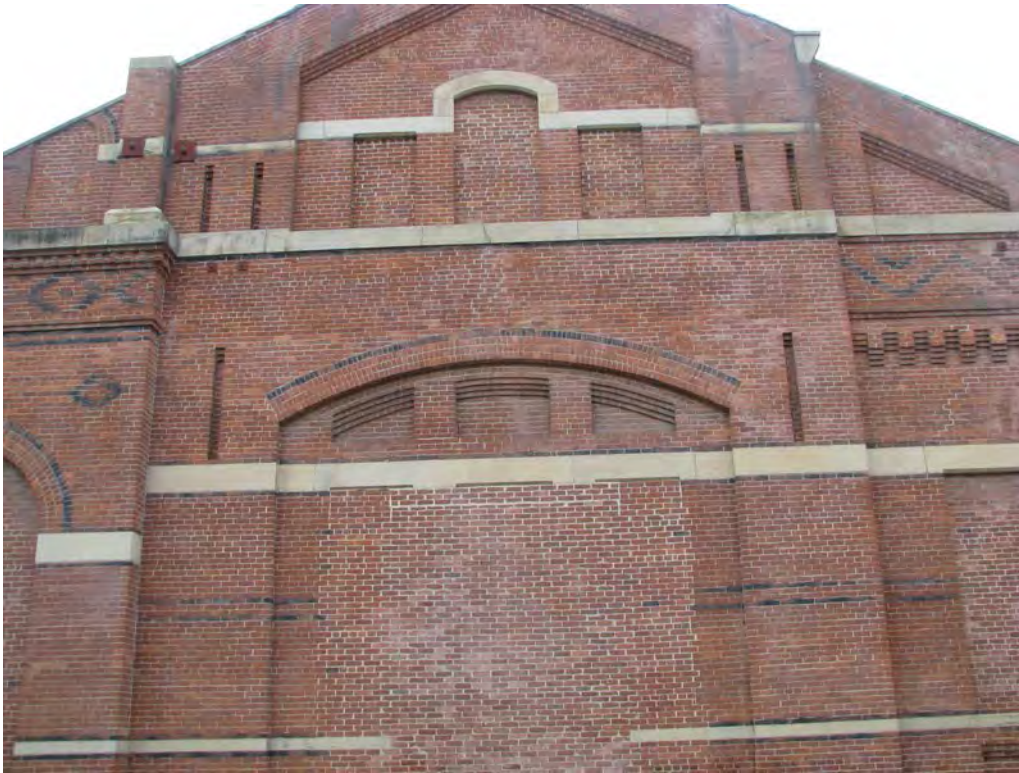
Photo 393 2817 Riverside Drive- Duke Energy (formerly Cincinnati Gas and Electric)
