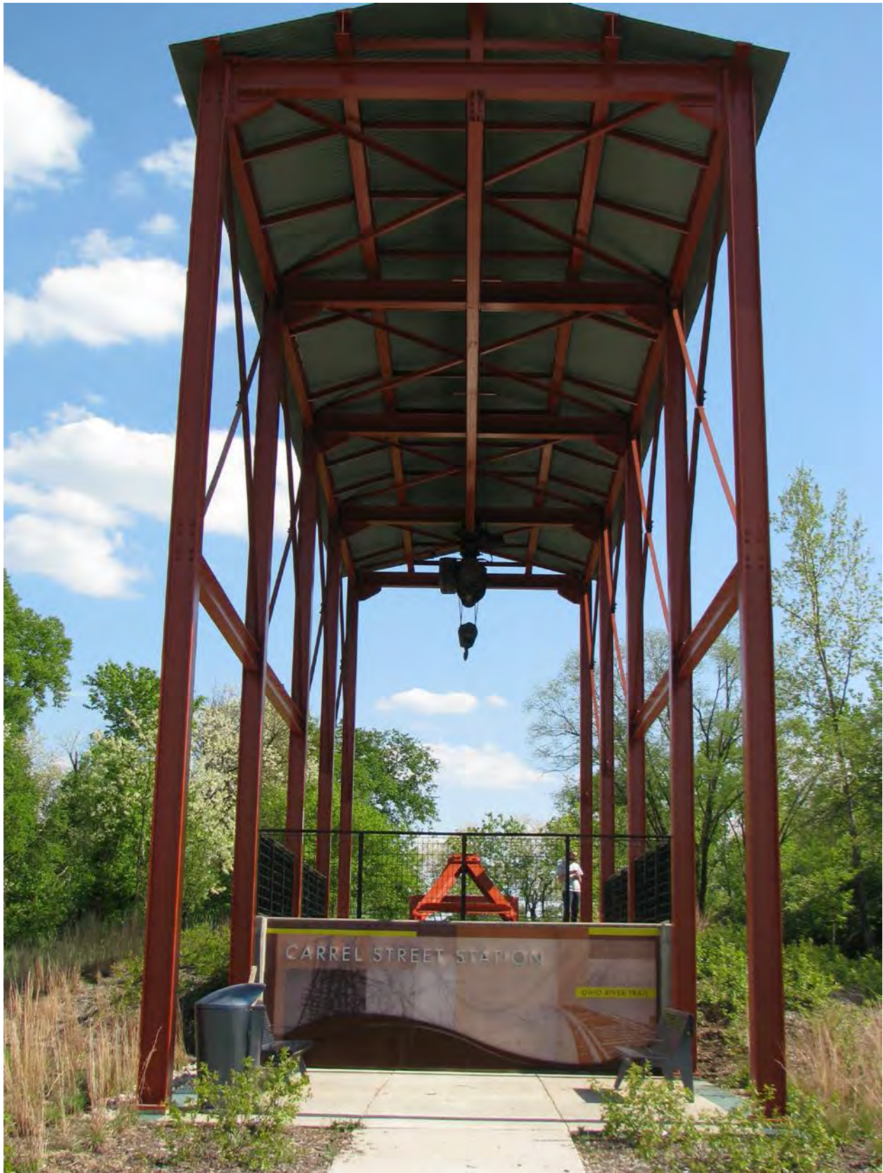
Photo 389 Carrel Street Station Train Winch
