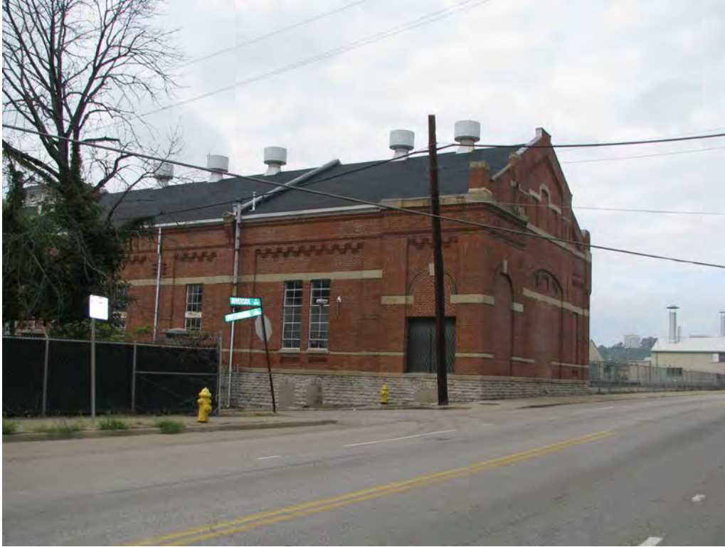
Photo 391 2817 Riverside Drive- Duke Energy (formerly Cincinnati Gas and Electric)
