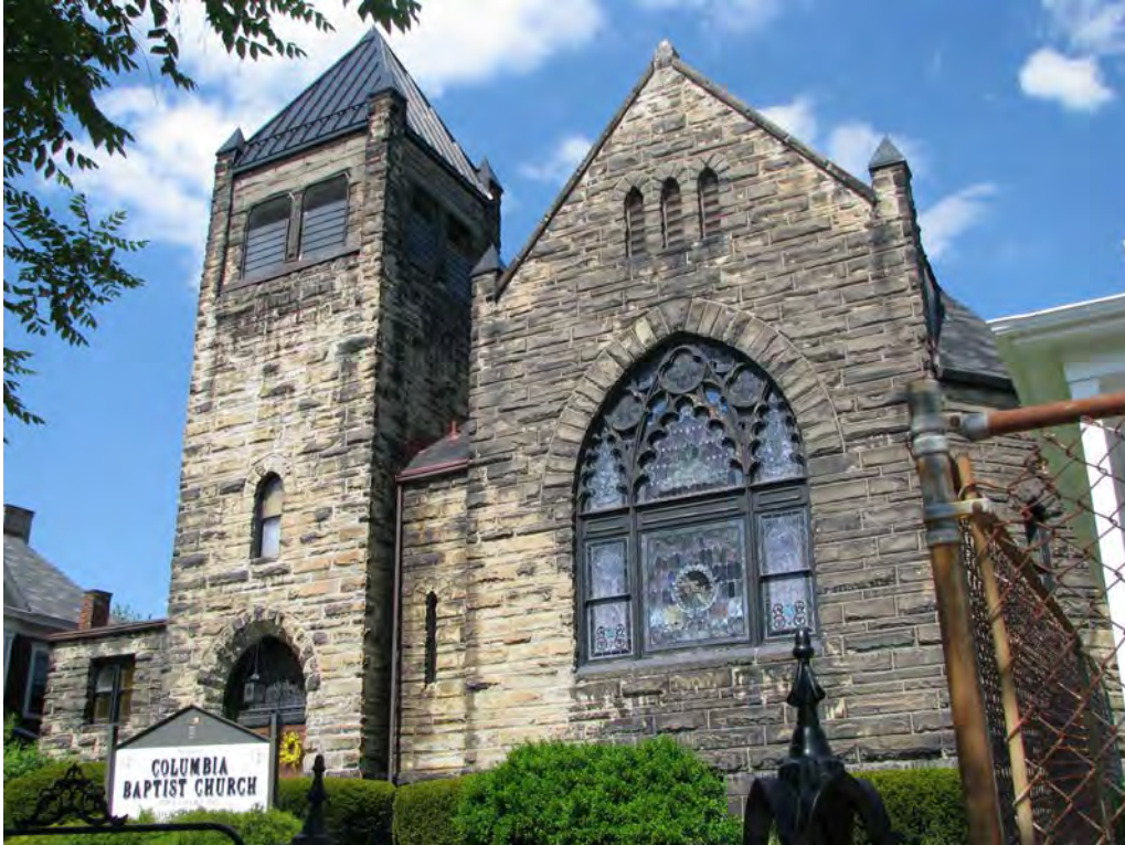
Photo 357 3718 Eastern Avenue- Columbia Baptist Church (part of NR#79002699)
