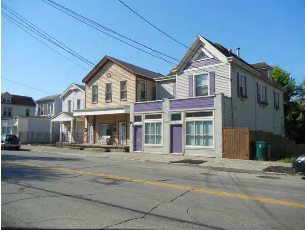
Photo 376 3729 and 3731 Eastern Avenue
