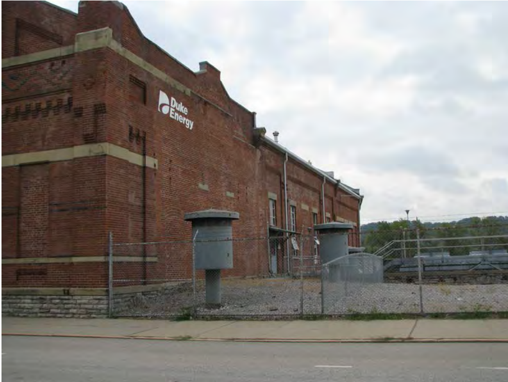
Photo 392 2817 Riverside Drive- Duke Energy (formerly Cincinnati Gas and Electric)
