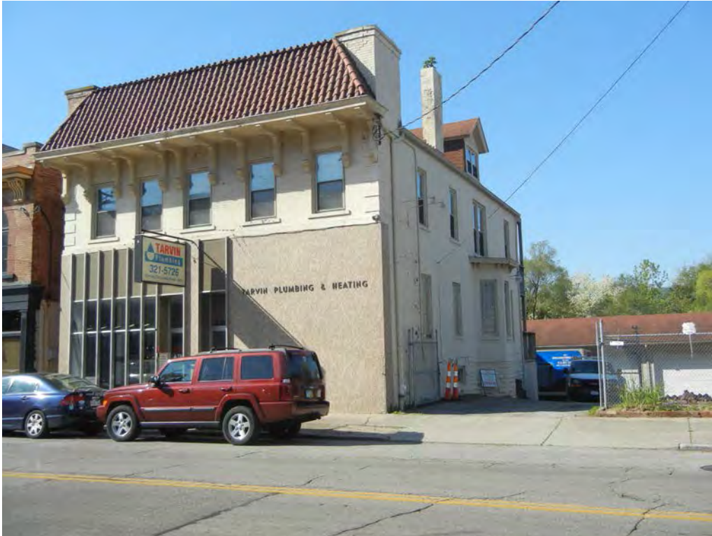
Photo 379 3747 and 3749 Eastern Avenue
