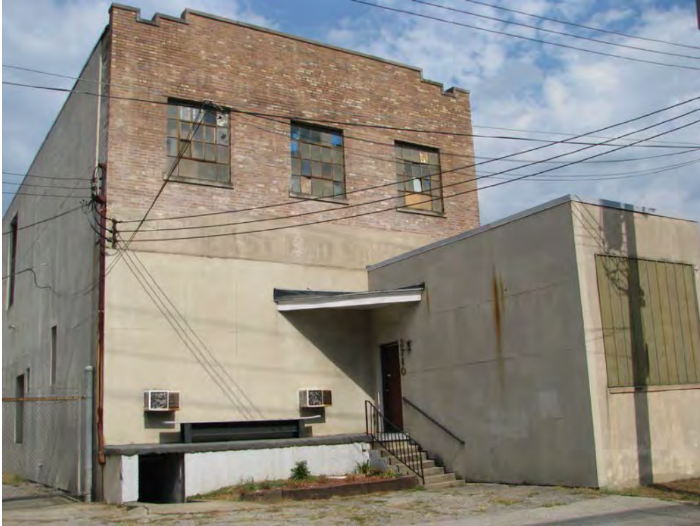
Photo 260 3710 Beechmont Avenue-“East End Supply”
