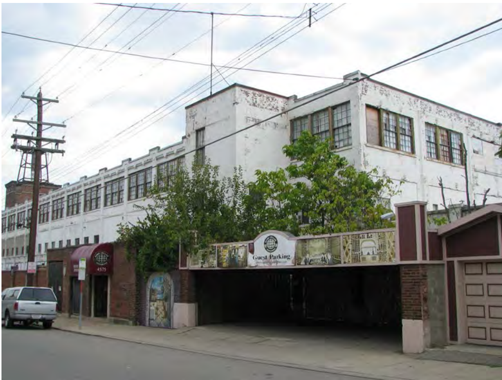
Photo 257 4575 Eastern Avenue- "Wine Cellar"
