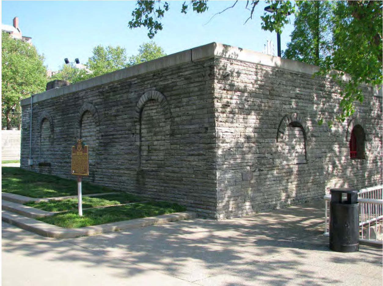
Photo 388 Pumping Station in Sawyer Park (HAM-2012-17)
