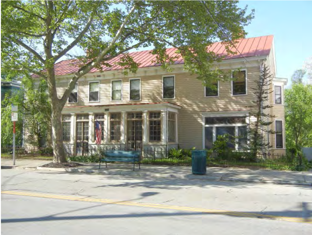
Photo 383 3807 and 3811 Eastern Avenue (part of NR#79002699)
