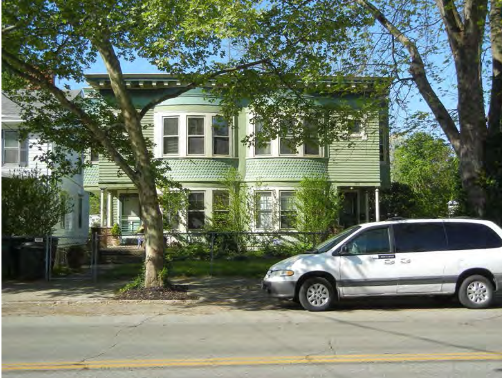
Photo 384 3815 and 3817 Eastern Avenue (part of NR#79002699)
