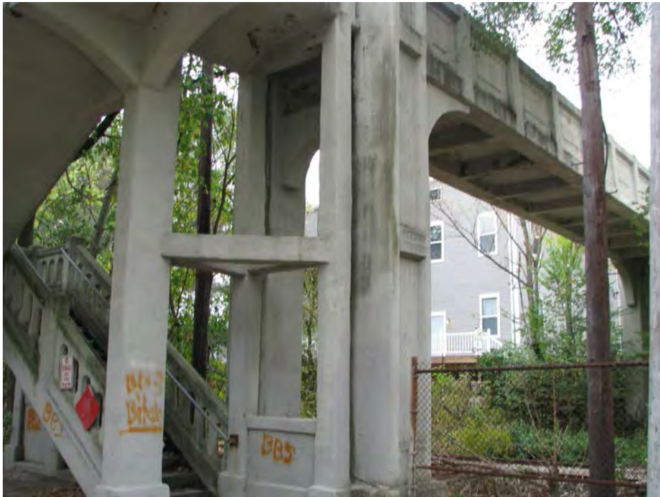
Photo 291 Stone steps and walk path connecting Greenwood Terrace and Eastern Avenue-crosses tracks
