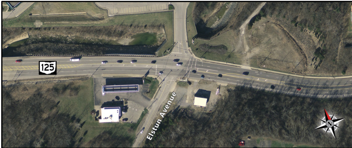
Figure 28. SR 125/Elstun Road Intersection
